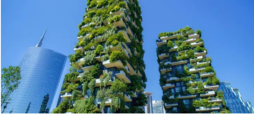
Figure 15: Building in Milano, named “Bosco Verticale” | Source
