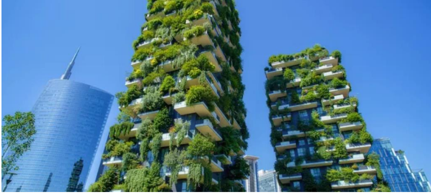
Figure 15: Building in Milano, named “Bosco Verticale” | Source
